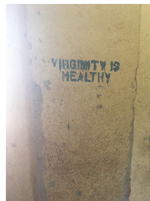
Messages spray painted onto classroom walls
